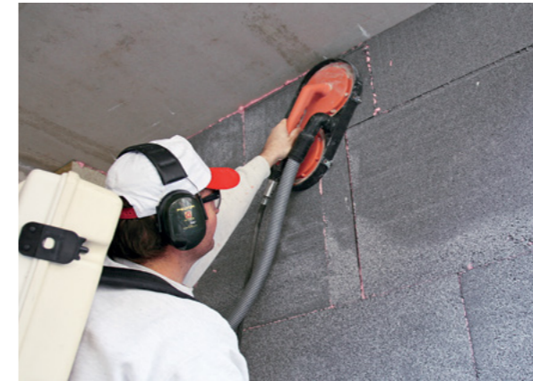
Grinding EIFS and ETICS boards
