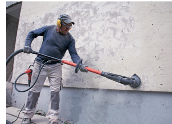
Removing old plaster and paints
