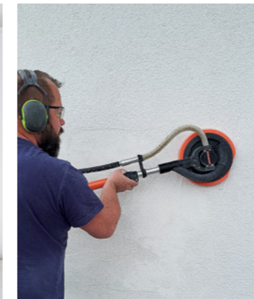
Removing plaster with a PCD disc
