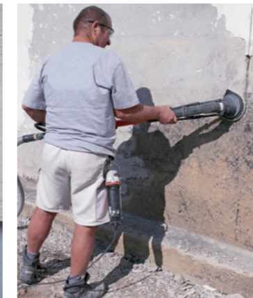
Grinding bitumen coating with PCD grinding disc
