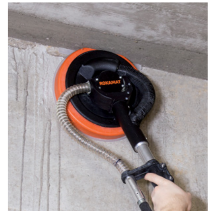
Grinding concrete burrs
