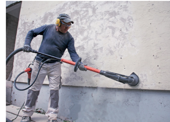
Removing old plaster and paints
