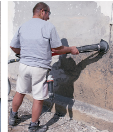
Grinding bitumen coating with PCD grinding disc
