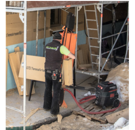
Side-mounted dust extraction
