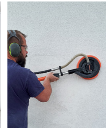
Removing plaster with a PCD disc
