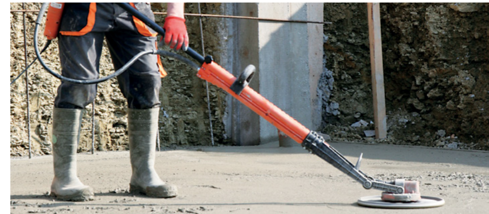
Levelling fresh concrete
