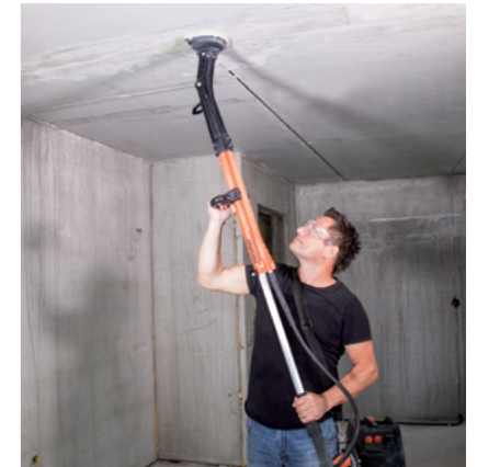
Ceiling grinding
