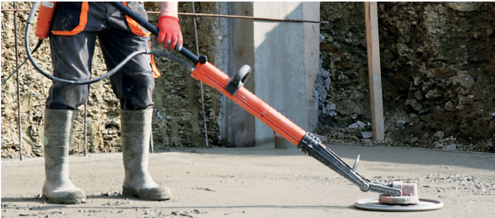
Levelling fresh concrete
