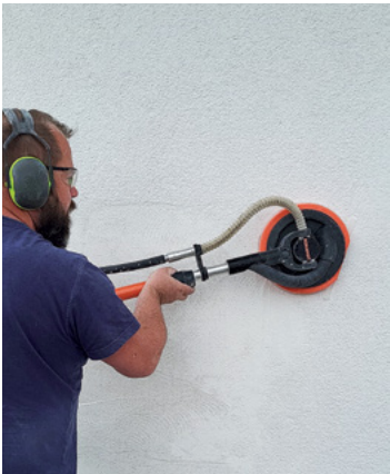
Removing plaster with a PCD disc
