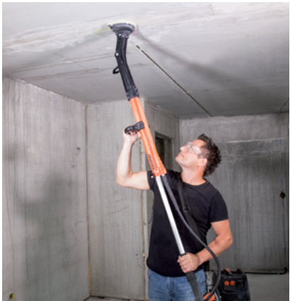
Ceiling grinding
