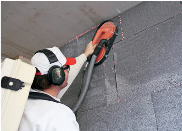
Grinding EIFS and ETICS boards
