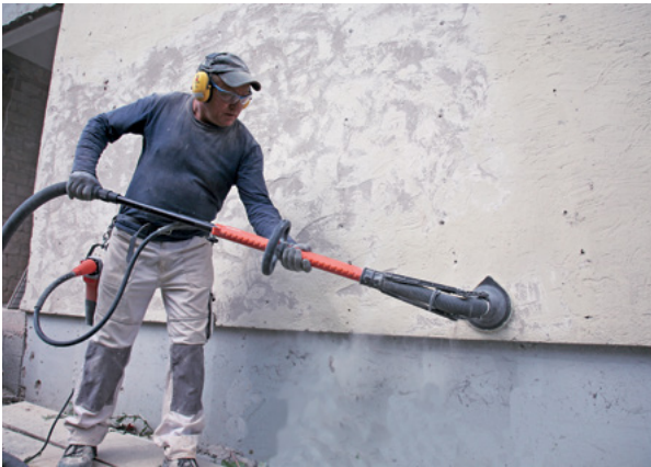
Removing old plaster and paints
