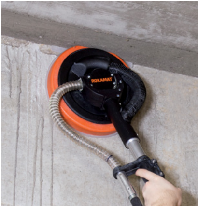
Grinding concrete burrs
