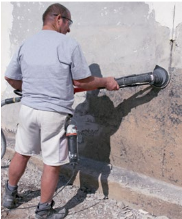
Grinding bitumen coating with PCD grinding disc
