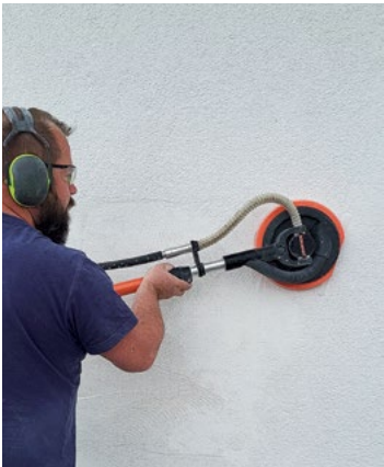
Removing plaster with a PCD disc
