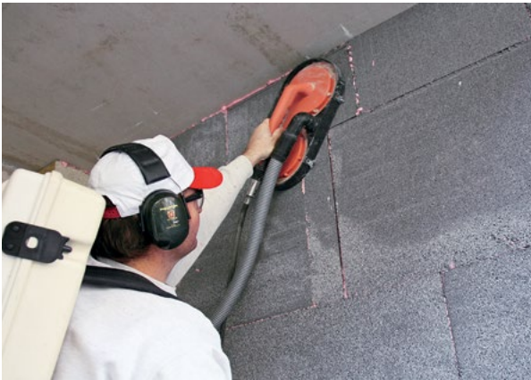
Grinding EIFS and ETICS boards
