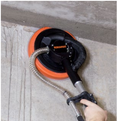
Grinding concrete burrs
