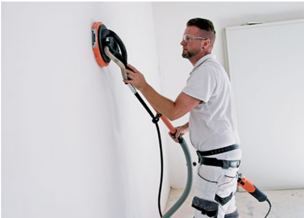
Grinding large surfaces very quickly
