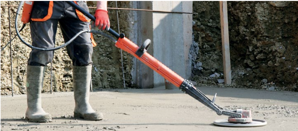
Levelling fresh concrete
