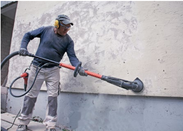
Removing old plaster and paints
