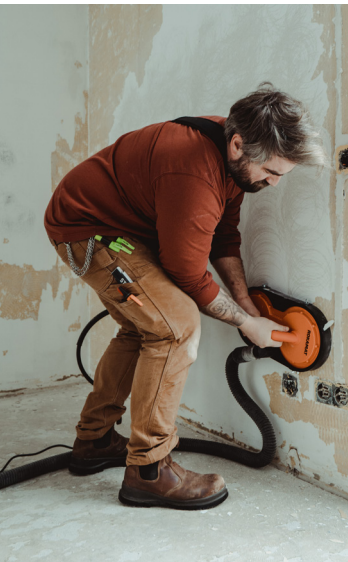
Removing old paint
