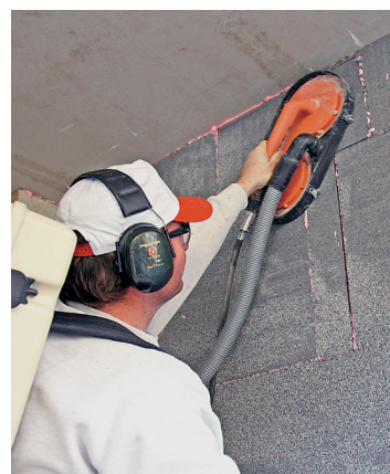
Grinding EIFS and ETICS boards
