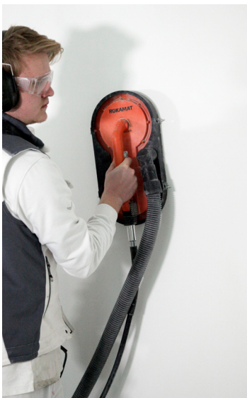
Grinding plaster
