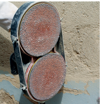
Aggressive grinding with metal abrasive discs
