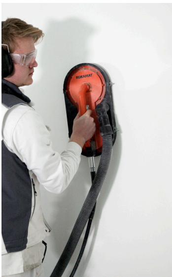
Grinding plaster
