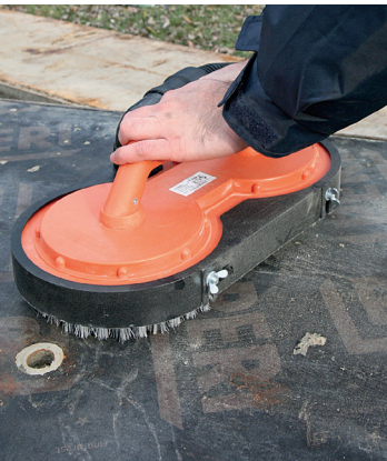
Cleaning formwork units
