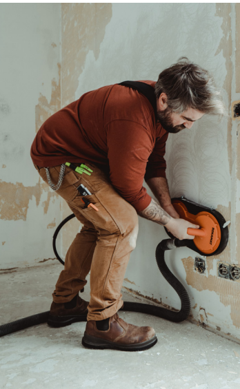
Removing old paint
