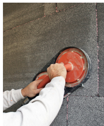
Grinding EIFS and ETICS boards
