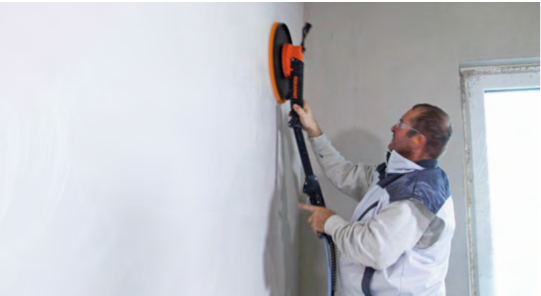
Sophisticated engine technology: Lower rotation speed possible → for a perfect surface structure
