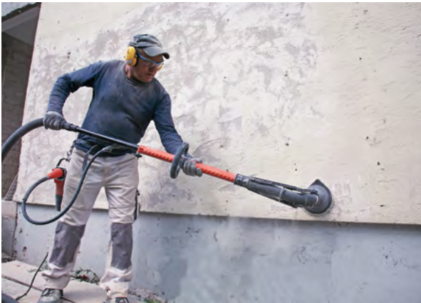
Removing old plaster and paints
