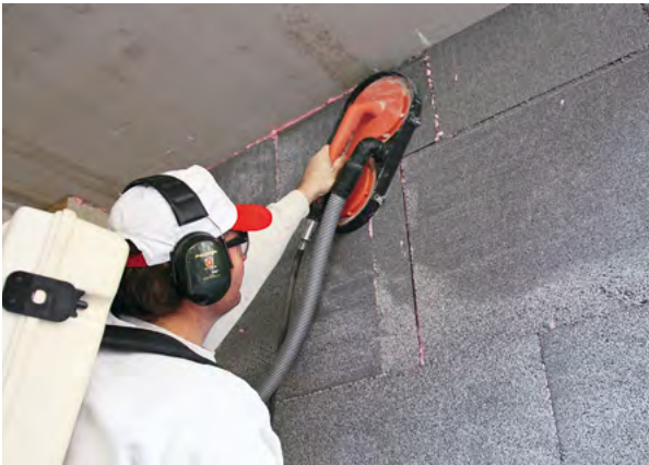
Grinding EIFS and ETICS boards
