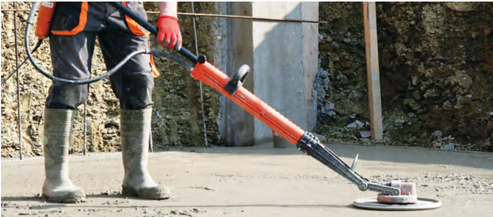
Levelling fresh concrete
