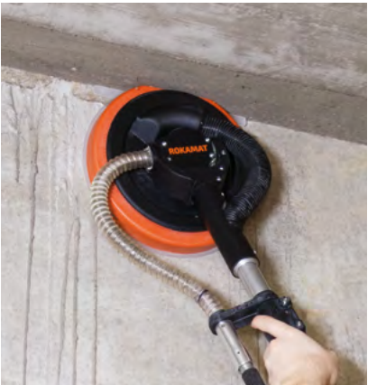
Grinding concrete burrs
