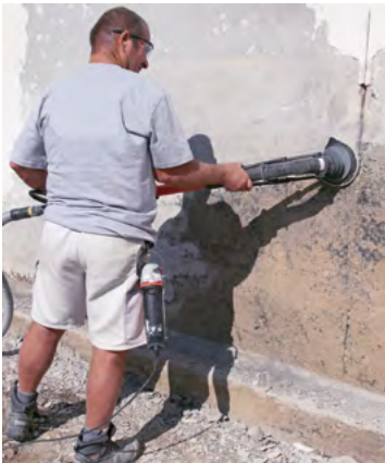
Grinding bitumen coating with PCD grinding disc
